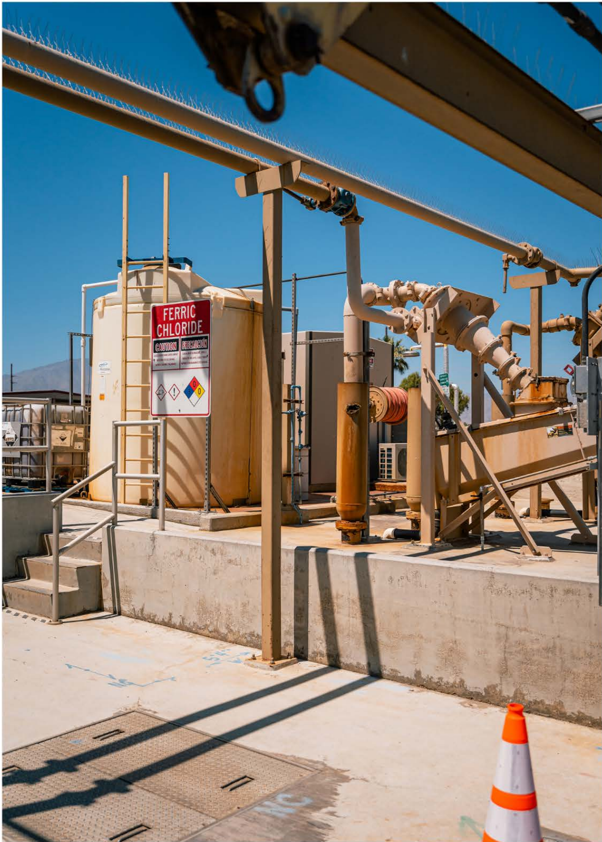
Ferric Chloride Tank
