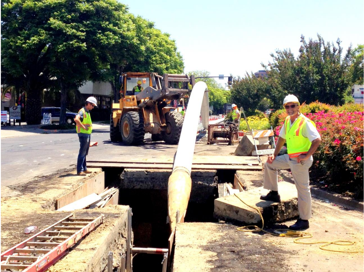
Example of Pipe Busting 10 inch ID VCP with 20 inch OD HDPE
