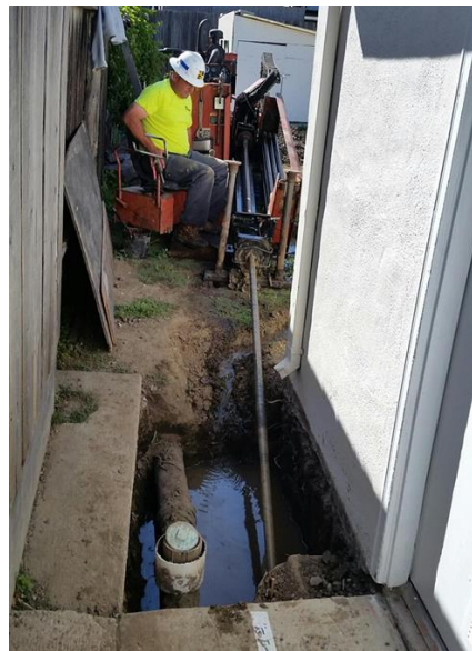
Photos of sewer lateral rerouting from backyards to the new sewer main in the street
