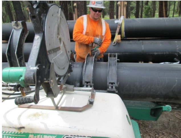
Figure 3: Fusion welding
