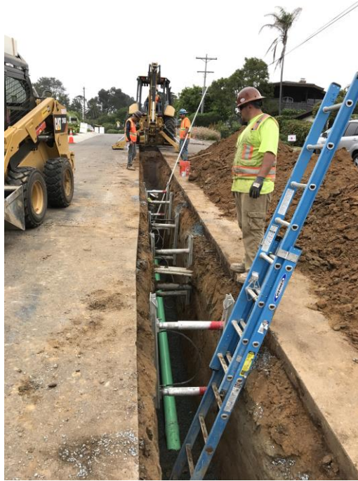
6-Inch Sewer Open Trench Installation
