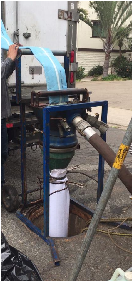
Example of CIPP Installation
