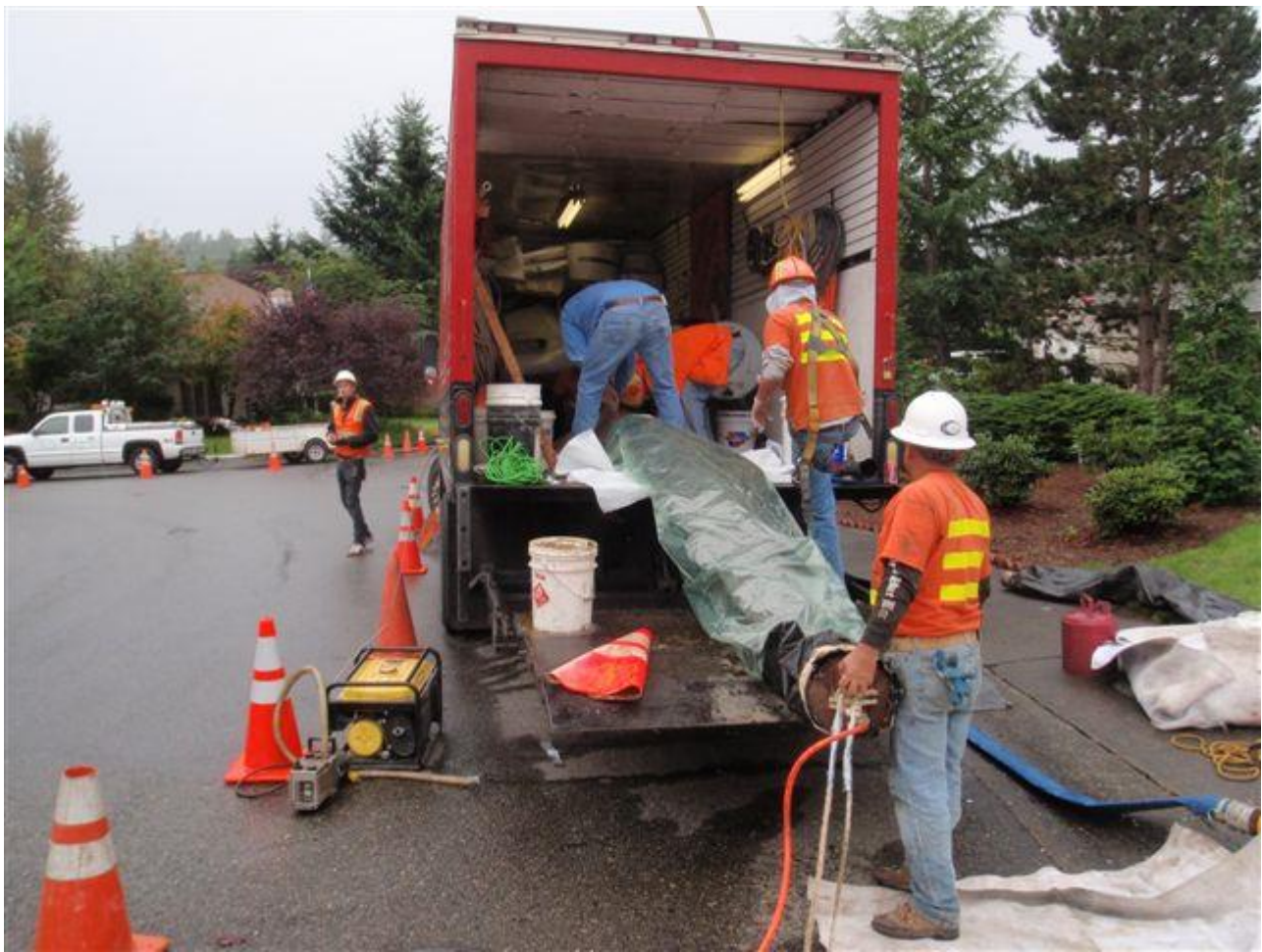
15-inch diameter CIPP spot repair sleeve prepared onsite and ready for installation
